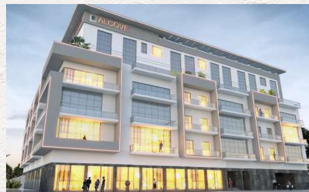
ALCOVE, JVC completed 2016 www.grovy.ae/alcove
